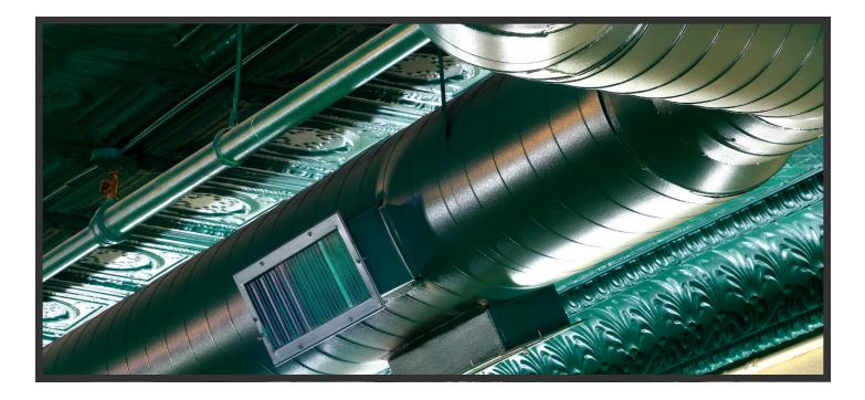
Both pressure drop and velocity decrease as the cross-sectional area of a duct becomes larger, but there is an upper limit to how much duct size can be increased.
