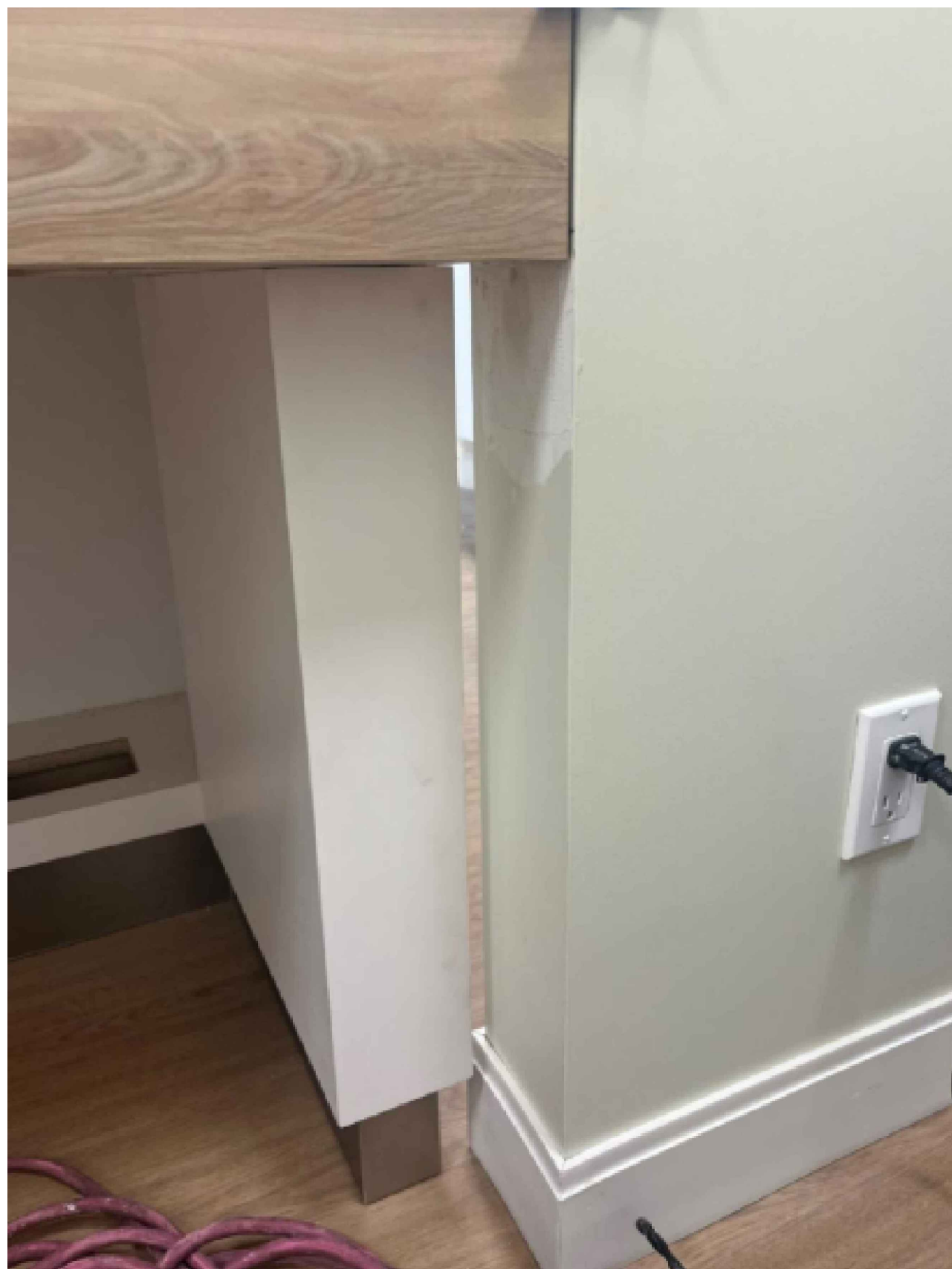
10 FINAL RECEPTION DESK INSTALLATION. NO WIRING EXPOSED NOTE THE RELATIONSHIP BETWEEN DESK LEG TO WALL
