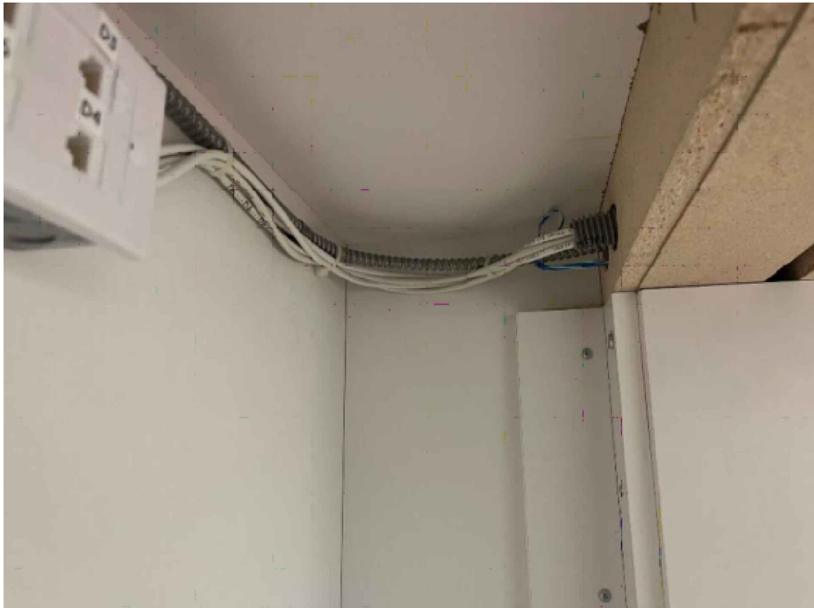
9 DATA AND POWER FEED ENTERING FRONT OF WHITE DESK CARCASS
