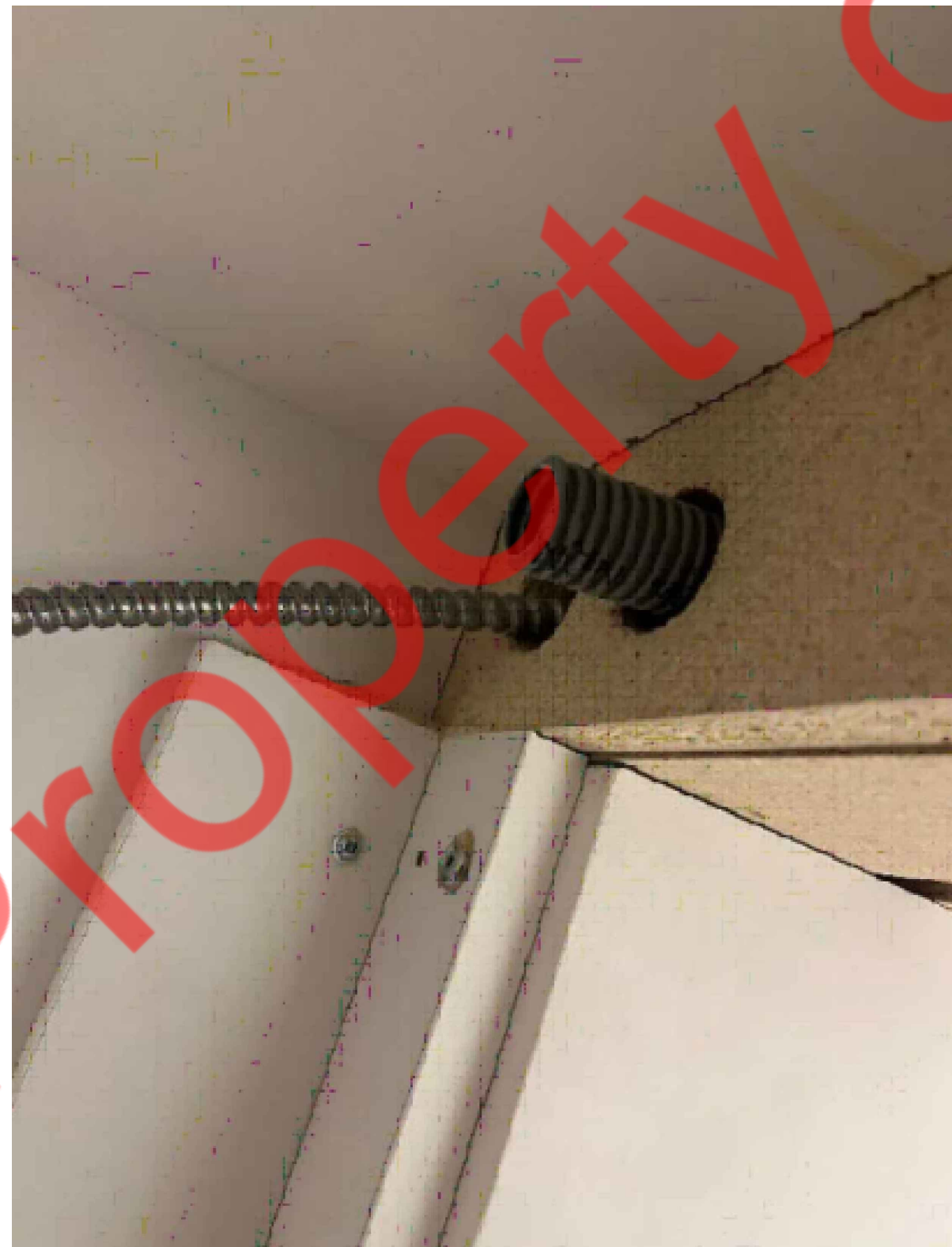
8 DATA AND POWER FEED ENTERING FRONT OF WHITE DESK CARCASS
